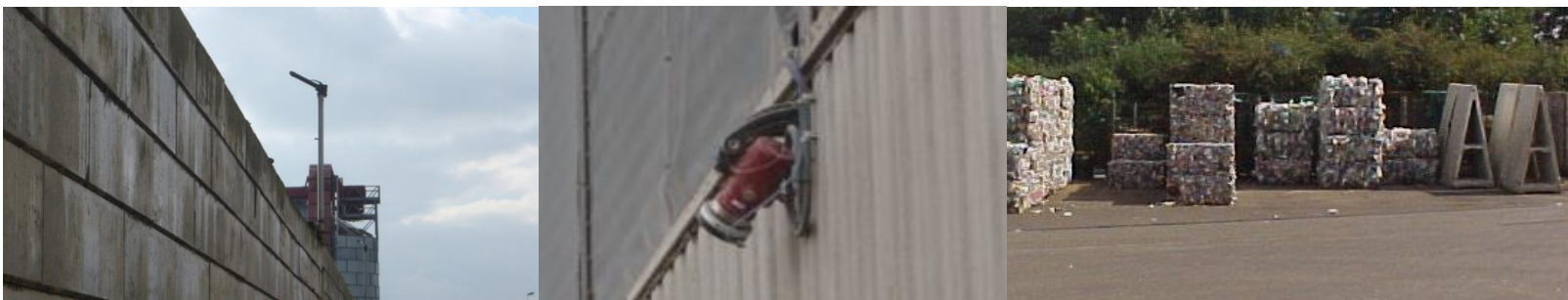
From left: Water deluge head mounted above external waste storage bunker wall (example only – deluge etc systems can be mounted lower or direct on walls), camera-type detector in external use above a waste bunker, standard bale storage ('A' frames in place for use as fire walls as required)
