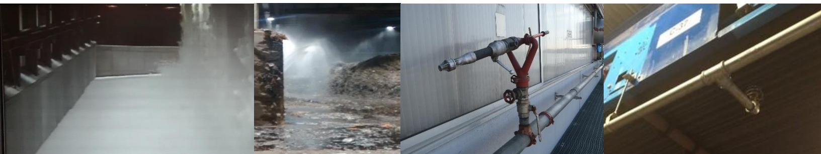
Left to right: Large foam system under test at a waste recovery plant, sprinklers in action at a recycling plant, manual-use water monitor at a waste site, under-gantry sprinkler head and pipework at a recycling plant
